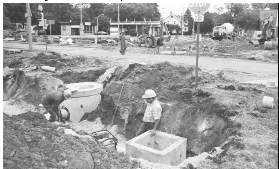
July 1988 - Sewer and road reconstruction work continues on Talbot St. W. with this photo capturing work done in front of the First Baptist Church at the corner of Talbot, Fox and Albert St.
